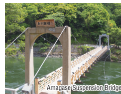
Amagase Suspension Bridge
